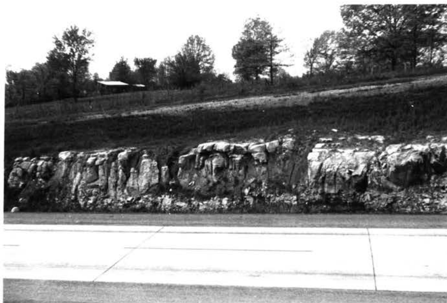
Fig. 17. Cutters and pinnacles in highway cut along the U.S. Highway 63 bypass at Thayer, Missouri.
